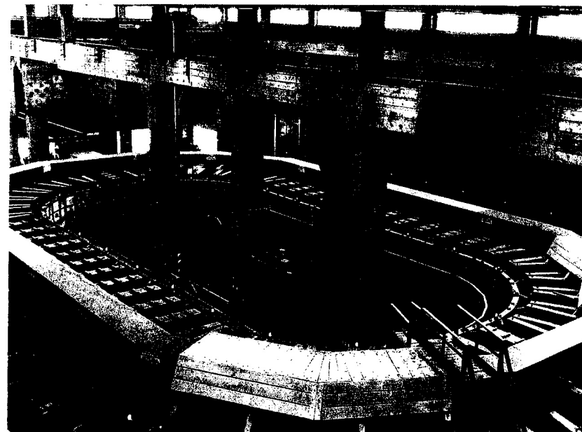
FIGURE 20.2 The Alpha-1 racetrack, Y-12 Plant in 1944. (U.S. Corps of Engineers, Manhattan Engineering District, Oak Ridge, Tennessee. Photograph by James E. Westcott). The Alpha-1 racetrack was used in the separation of uranium isotopes. This device gives some impression of the scale at which big science began to operate when the resources of the military-industrial complex were thrown behind it. The wiring used 6,000 tons of silver obtained from the U.S. treasury.
