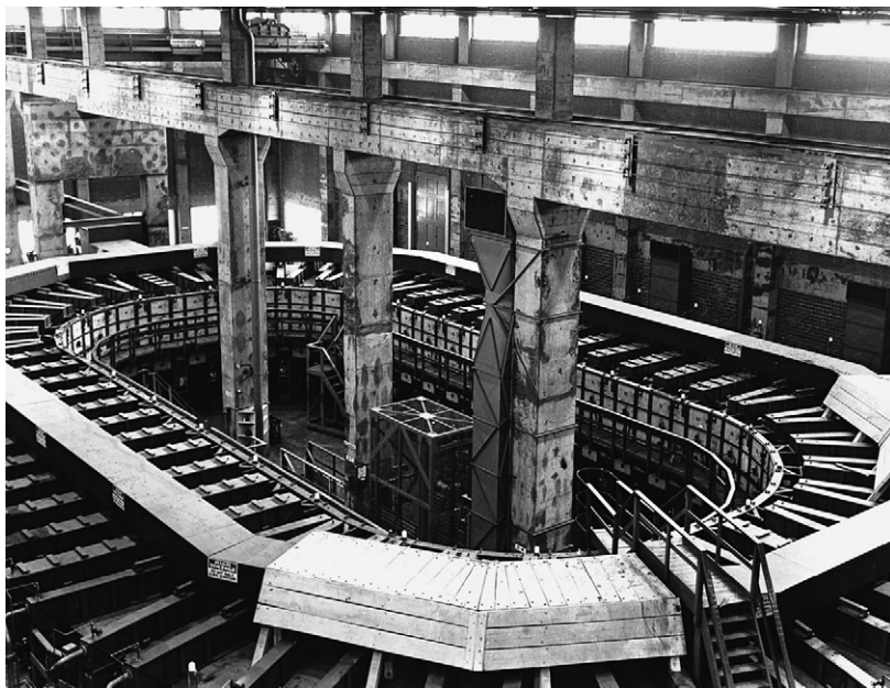
Fig. 21.2. The Alpha-1 racetrack, Y-12 Plant in 1944. US Corps of Engineers, Manhattan Engineering District, Oak Ridge, Tennessee. The Alpha-1 racetrack was used in the separation of uranium isotopes. This device gives some impression of the scale at which big science began to operate when the resources of the military-industrial complex were thrown behind it. The wiring used six thousand tons of silver obtained from the US Treasury. Photo by James E. Westcott.
